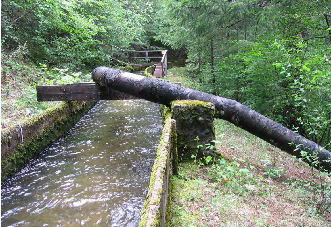
Photograph 2.2.2-1e South Canyon Creek – Canal Siphon Release To Kilarc Main Canal
