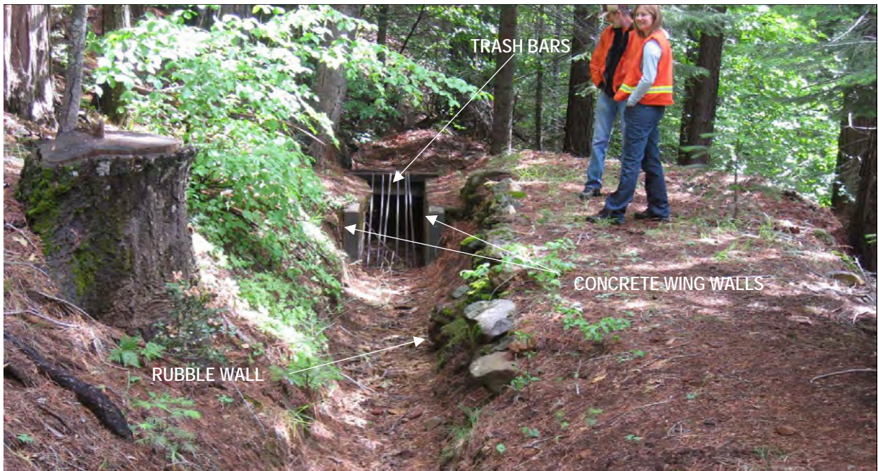
Photograph 2.2.2-1d South Canyon Creek – Canal Siphon Inlet
