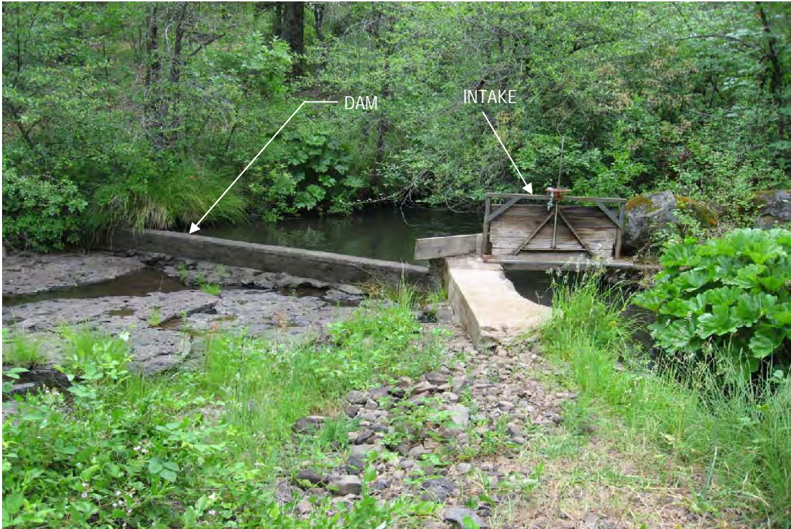
Photograph 2.3.1-1 Mill Creek Diversion – Dam and Canal Intake
