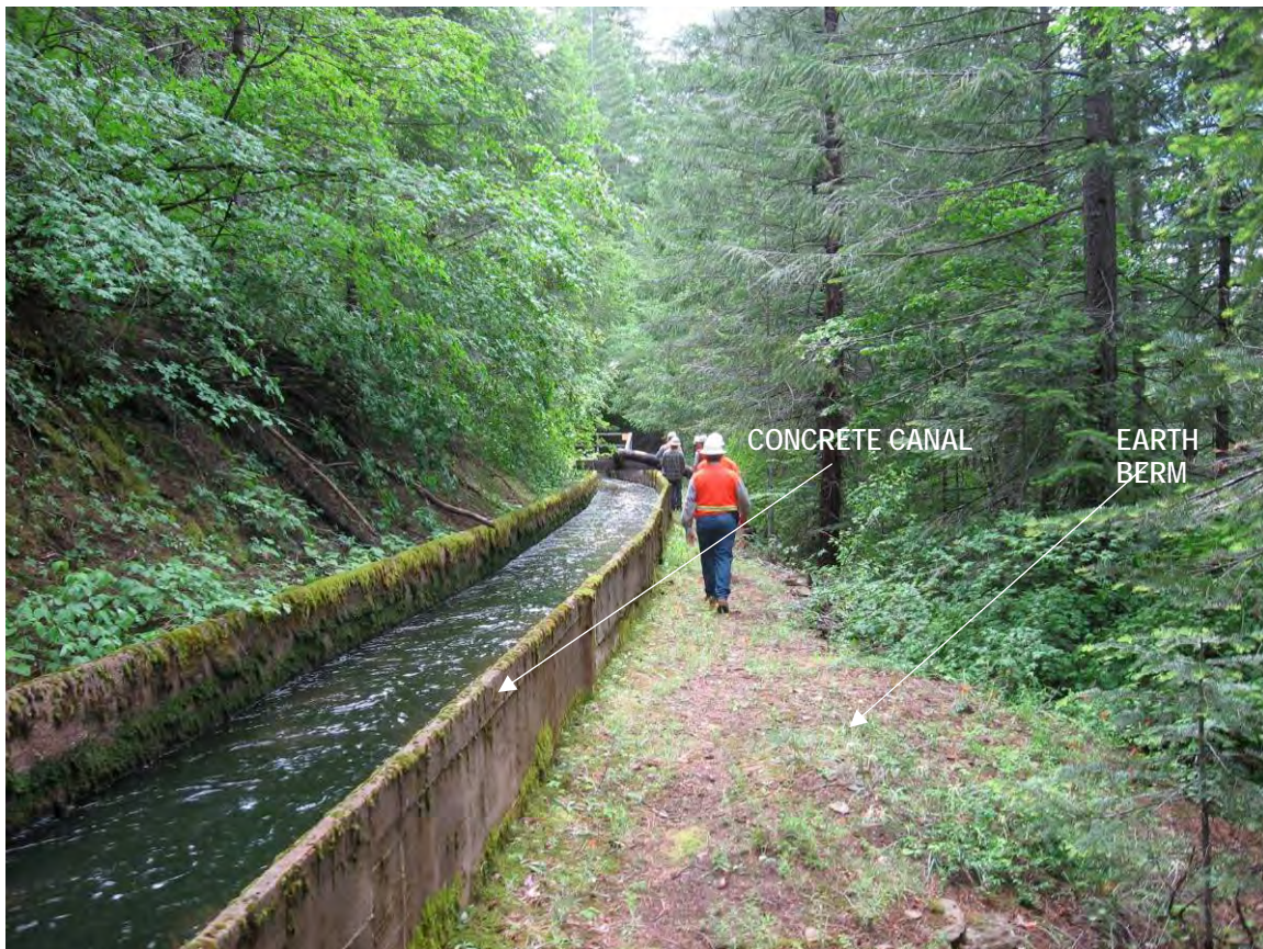
Photograph 2.2.4-1a Kilarc Main Canal – Concrete Section
