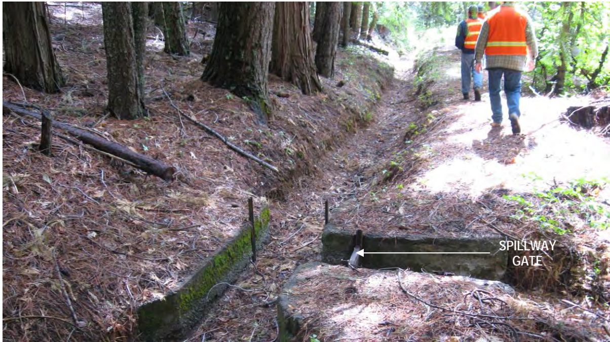
Photograph 2.2.2-1d South Canyon Creek – Canal Siphon Inlet
