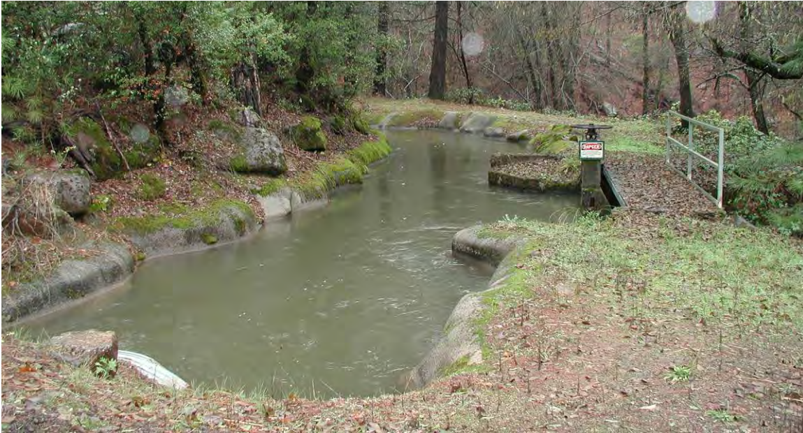
Photograph 2.3.4-1d South Cow Creek – Shotcrete Section
