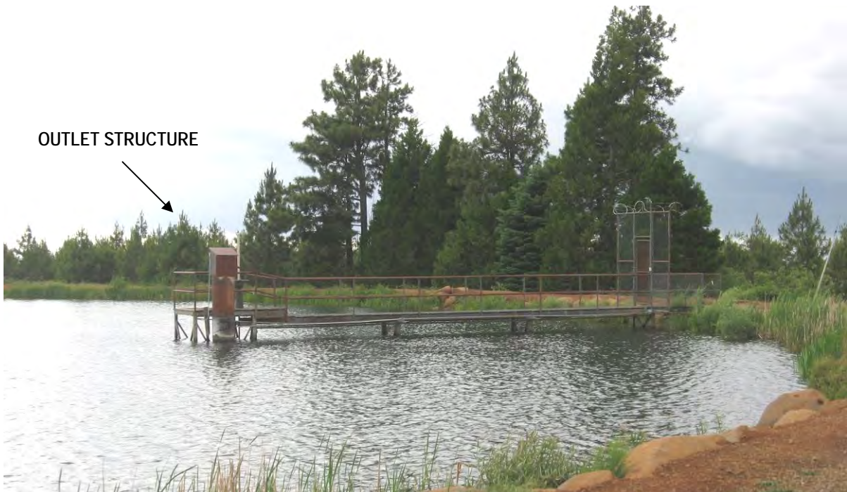
Photograph 2.2.5-1d Kilarc Forebay – Outlet Structure to Penstock
