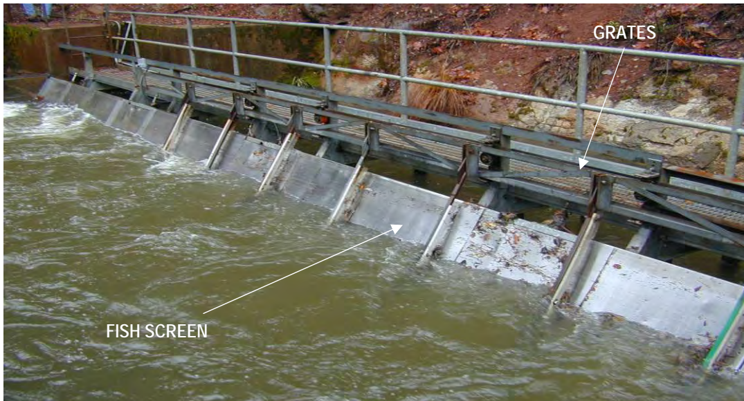
Photograph 2.3.3-1c South Cow Creek Diversion – Fish Screen Detail
