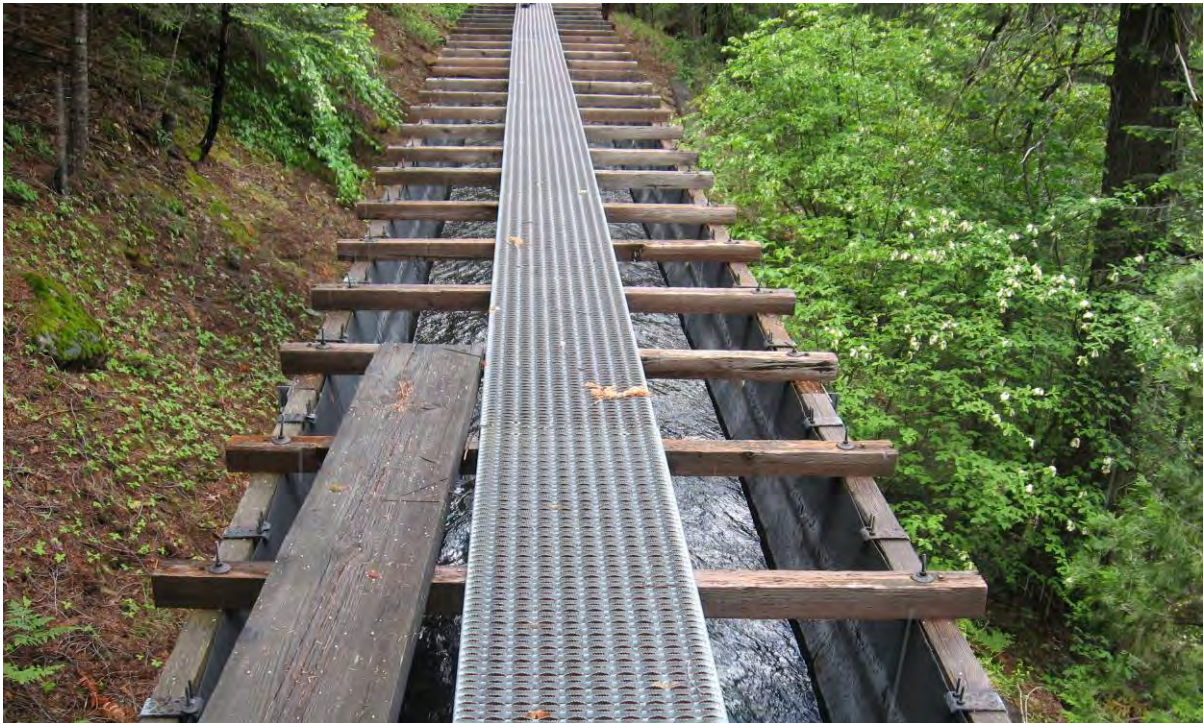
Photograph 2.2.4-1c Kilarc Main Canal – Wooden Flume
