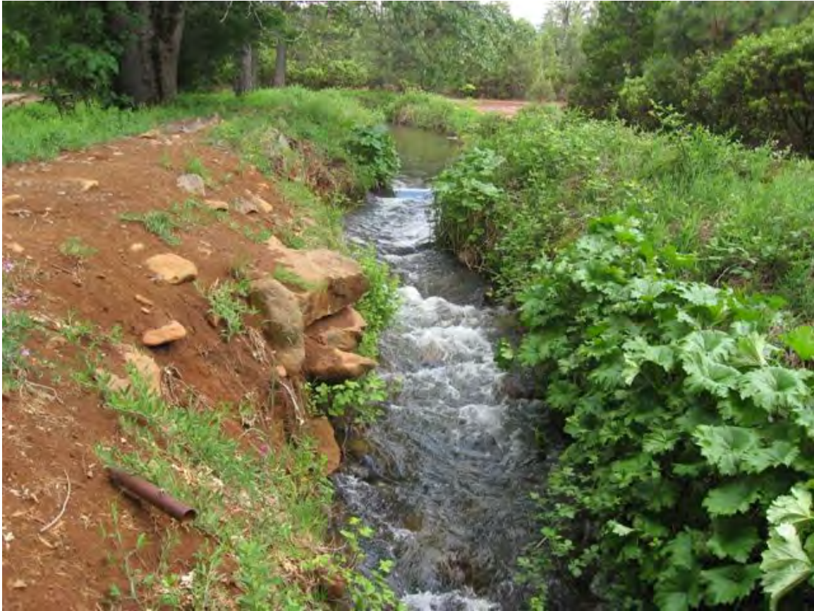
Photograph 2.2.4-1f Kilarc Main Canal – Earthen Section
